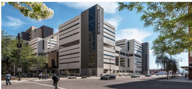
Photography by Mark Boisclair: Adaptive Reuse at 225 W. Madison, Formerly Madison Street Jail in Phoenix, AZ
