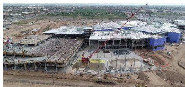
West Valley Casino Construction – back of house and parking structure
