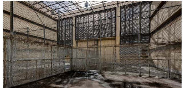
Courtesy of DLR Group: Madison Street Jail Inmate Recreation Yard (Before)
