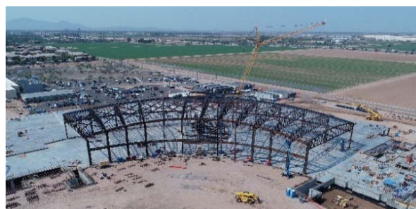
West Valley Casino Construction – Long Span Trusses
