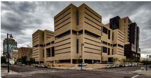
Courtesy of DLR Group: Madison Street Jail (Before)
