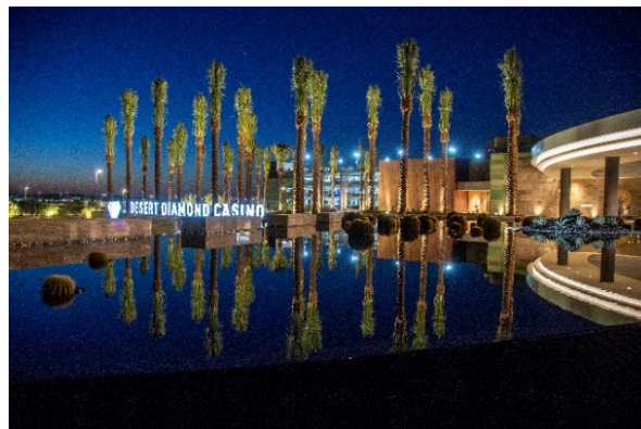
West Valley Casino Construction – finished entry view
