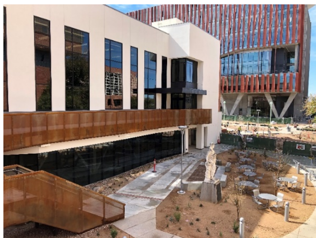
Skaggs North elevation looking west
