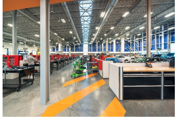
Discontinuous Diaphragm Due to Skylight in High Bay Roof
