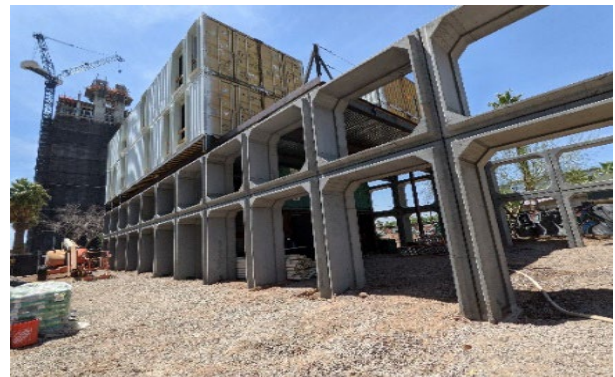
Setting Containers on the Culvert Structure
