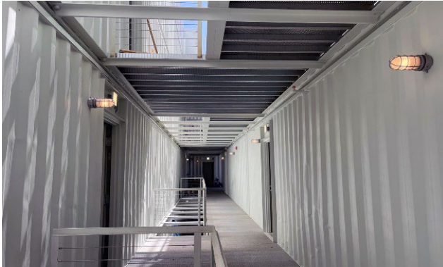
Open Structural Walkways for Water Collection
