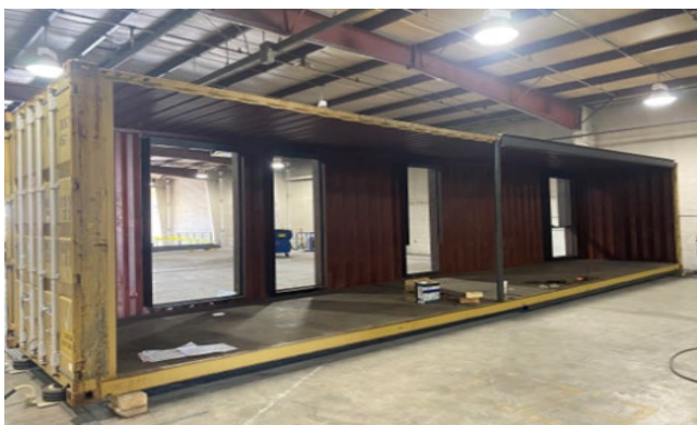
Container Fitup Prior to Placement
