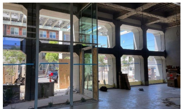
Glass Installation – Commercial Space
